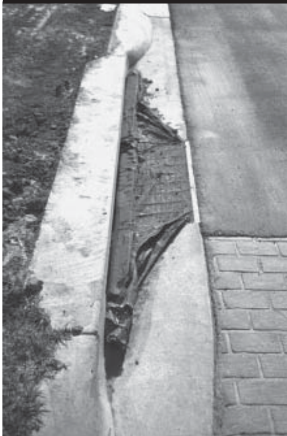
Plate 2.5 Stormwater Inlet Protection
