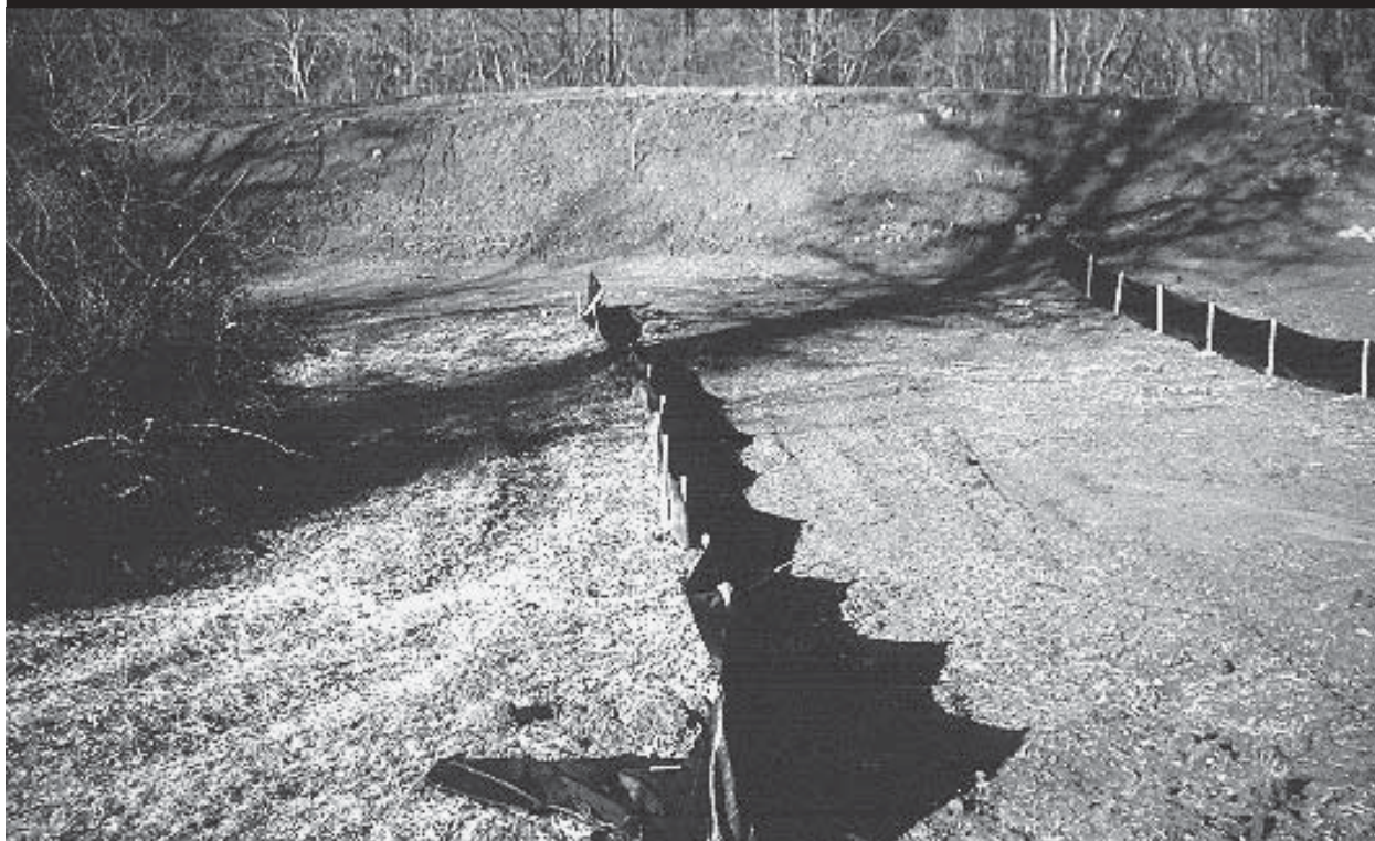
Plate 2.2 Silt Fence
